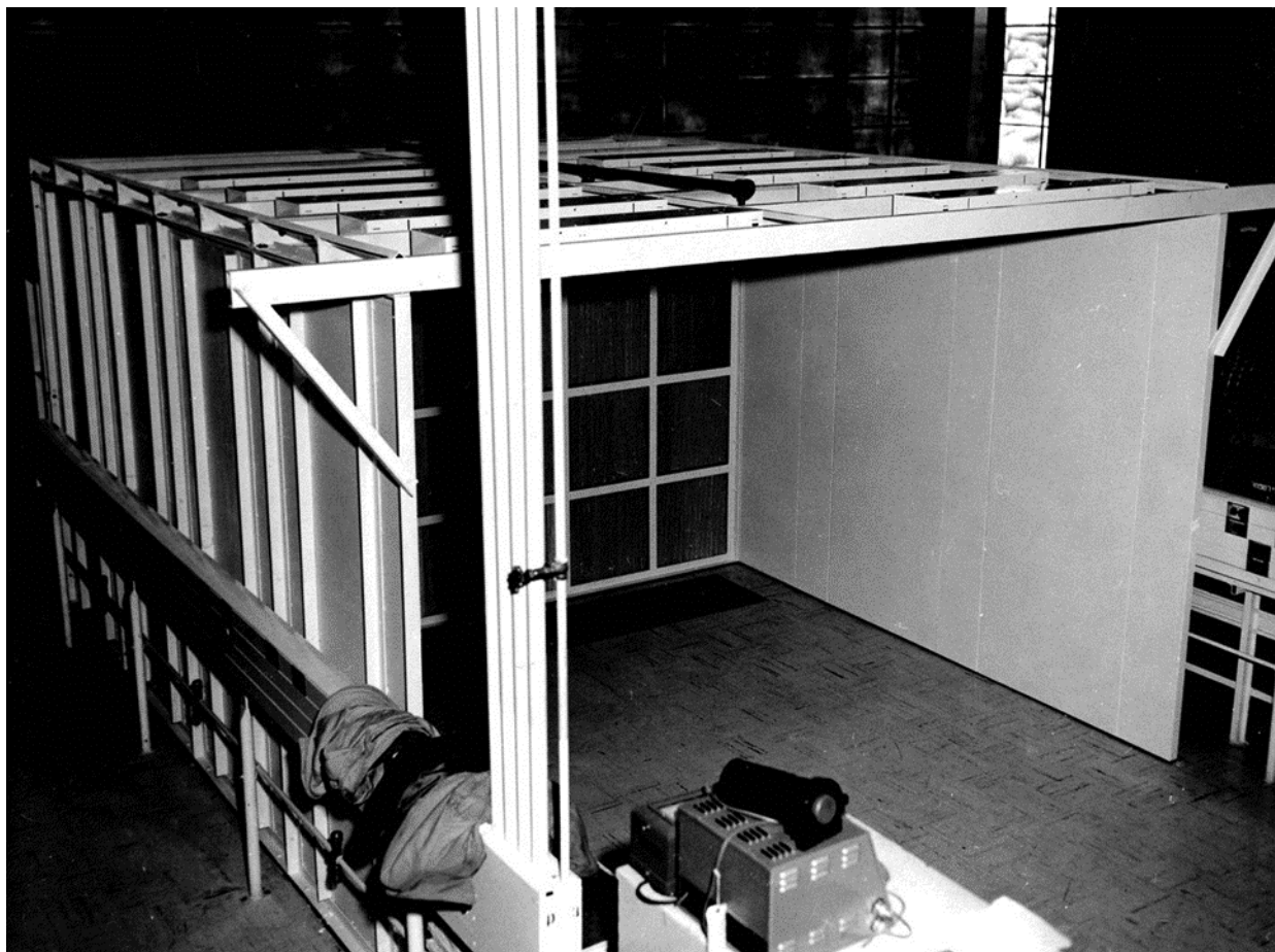
Figure 4. Completed Laminar Flow Tunnel. Robins AFB, Georgia. October 1962.
