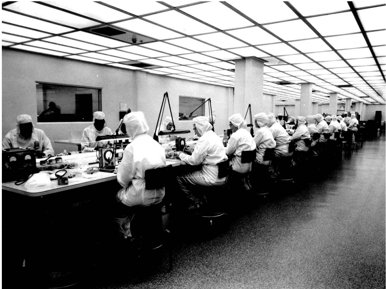
Figure 1. USAF Standard Class III Clean Room, Downflow. Robins AFB, Georgia. May 1962. (Return air at base of all four walls.)
