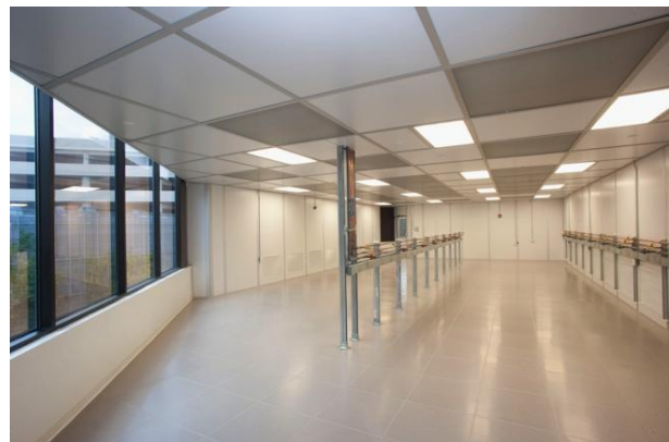
Figure 6—Finished Metrology Room ISO Class 6.
