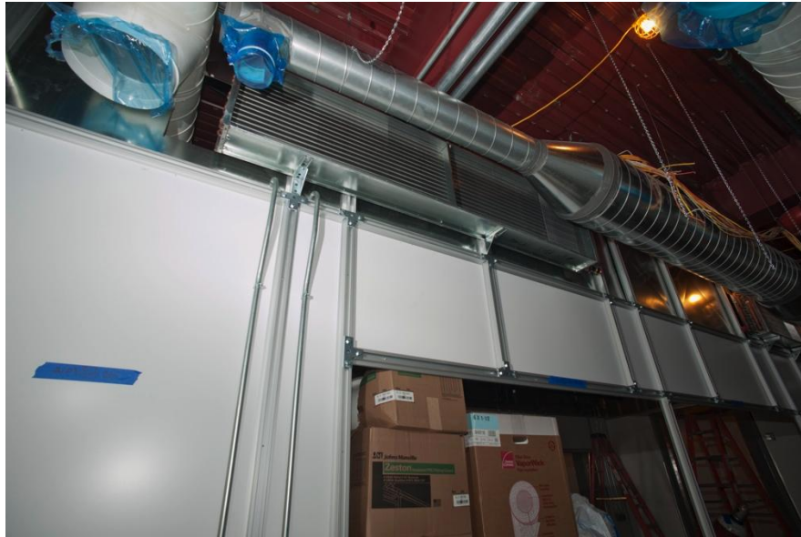
Figure 4—Installation of the sensible cooling coils and openings for tools.
