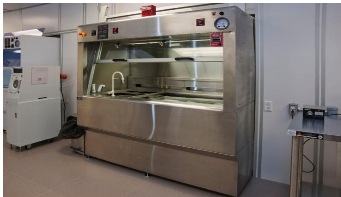
Figure 9—Typical wet bench installation.
