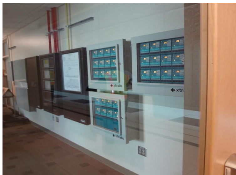
Figure 1. Example of an H5 Emergency Control Station (ECS).
